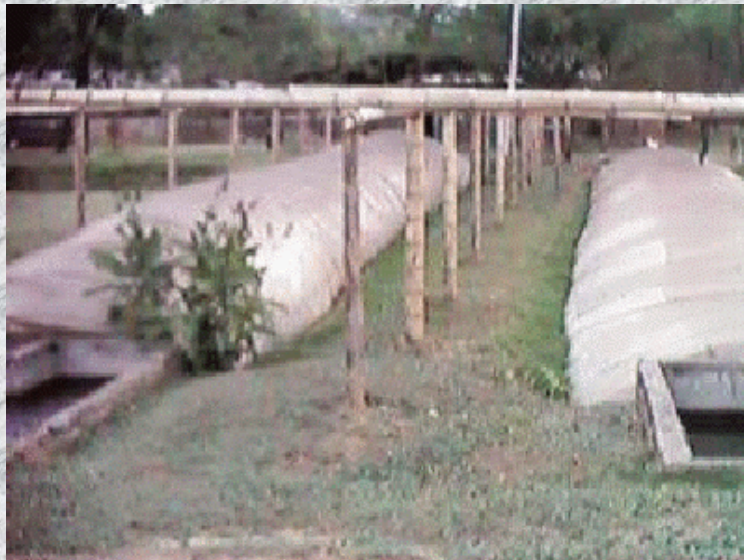
Plug Flow poly digesters
