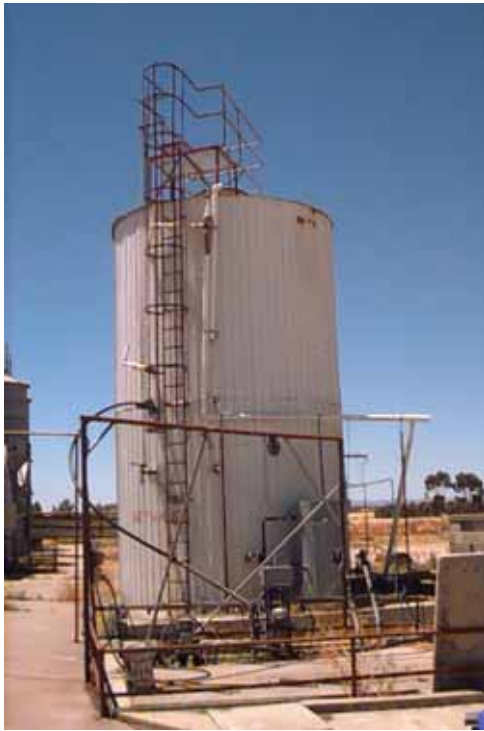
Fig 2 The CFST digester at Roseworthy Campus
