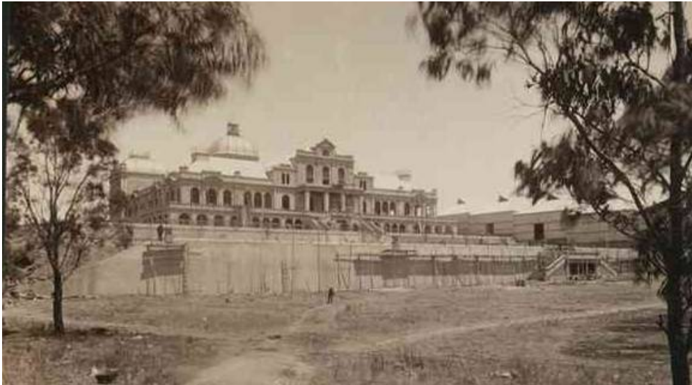
Exhibition Steps under construction in 1886 – lowest level on right.
