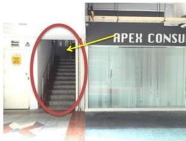
2. Beside 'Apex Consultant shop'
