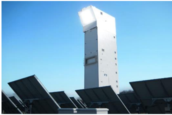
Figure 5: The demonstration of a solar thermal open volumetric air receiver (7.5 MW th ), heating air to 750 °C using DLR’s Solar Tower in Jülich, Germany (Sattler, 2018).
