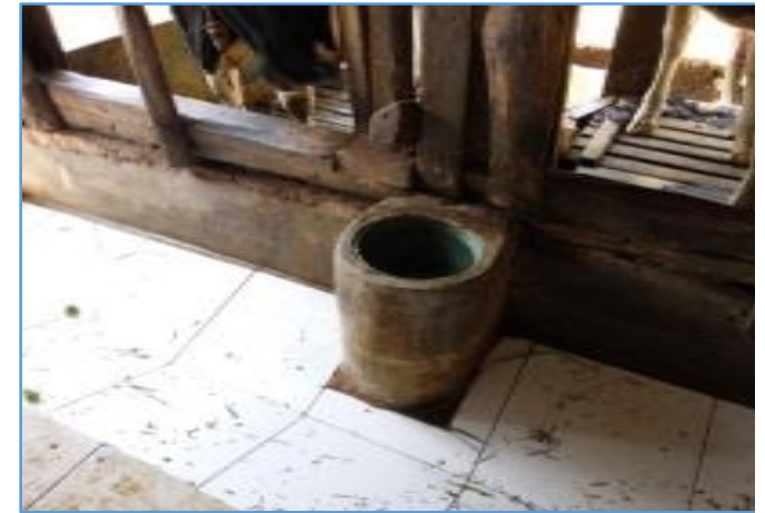
Adlibitum drinking water trough construction
