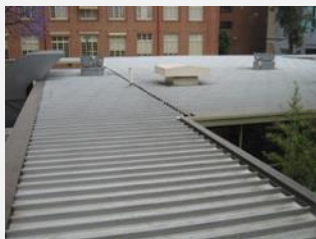
Lecture theatre roof
