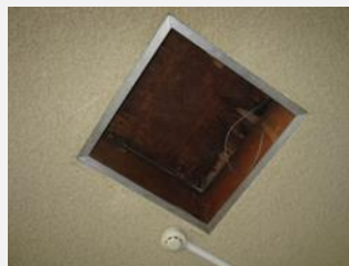
Access hatch to laboratory roof
