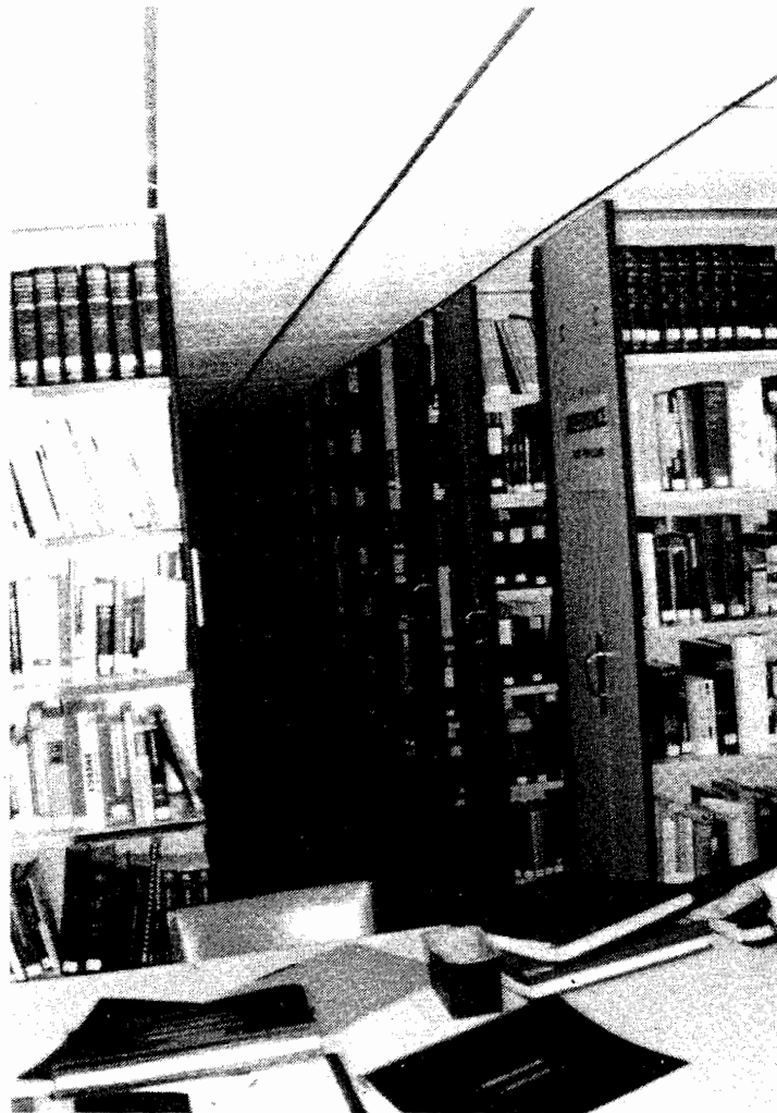
'The library building...suffered from several major faults'
