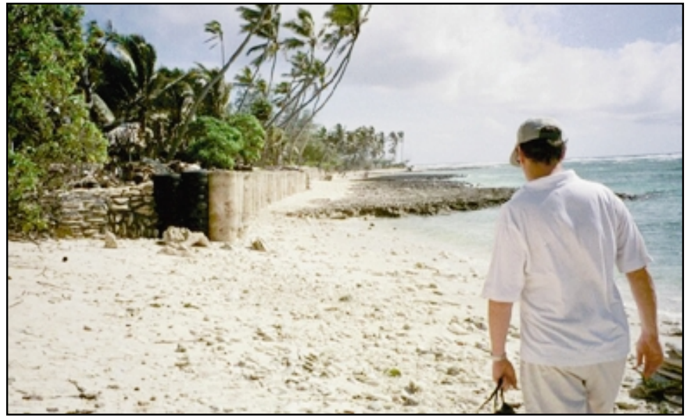
Dr Nick Harvey walks along a beach at Kiribati, where a concrete wall is all that stands between the sea and the atoll. Photo: Deirdre Hart.
