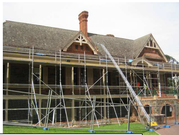
Restoration work on the northern side of Urrbrae House
