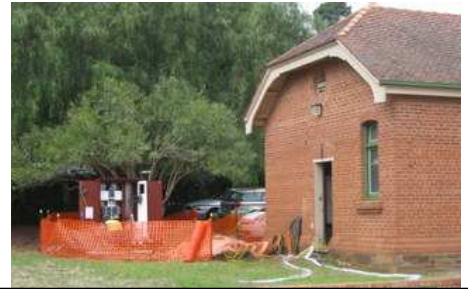
Resiting of the electrical switchboard from the battery house
