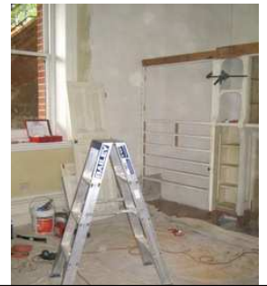
Carpentry work begins in the bedroom
